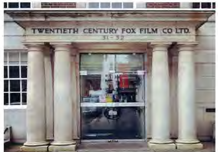
The Twentieth Century-Fox Film Co Ltd. Building Before its Demolition
